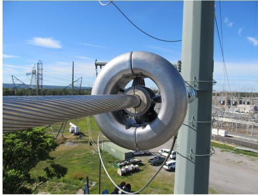
**Figura D.1:** Power Donuts de Usi-Power.
