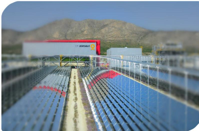
Figura 1.8: Colectores lineales Fresnel
