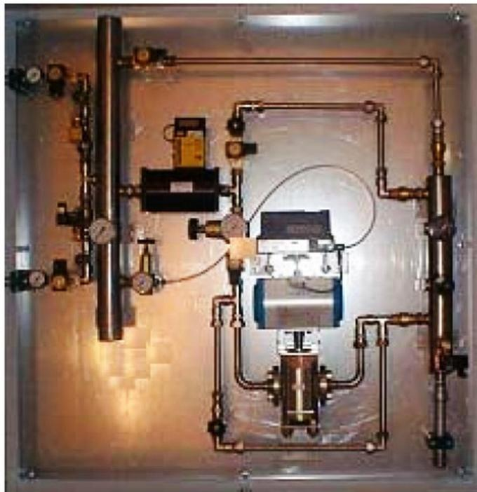
Gas Box with Real Flow Measurement and Control Valve
