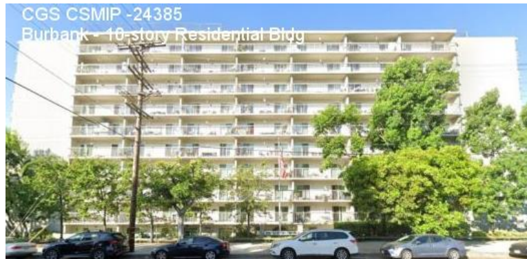
Figura 6: Edificio B158 “Burbank - 10-story Residential Bldg”, vista general.
