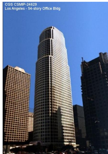
Figura 2: Edificio B205 “Los Angeles - 54-story Office Bldg”, vista general.
