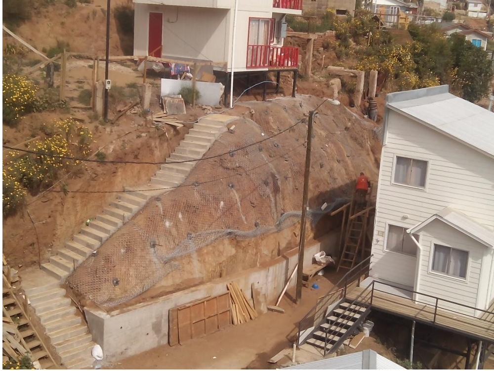
Figura 2-19. Vista general malla MFI3500-75 instalada shotcrete, TD N°88-2016
