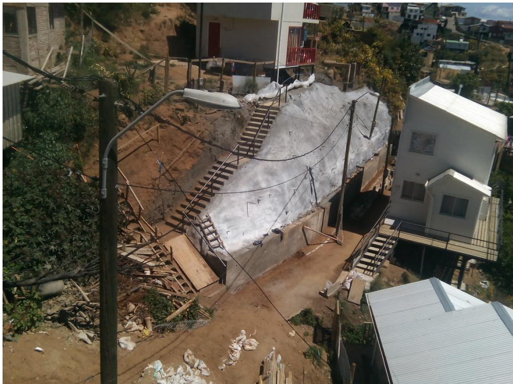
Figura 2-20. Vista general malla shotcrete terminado, TD N°88-2016
