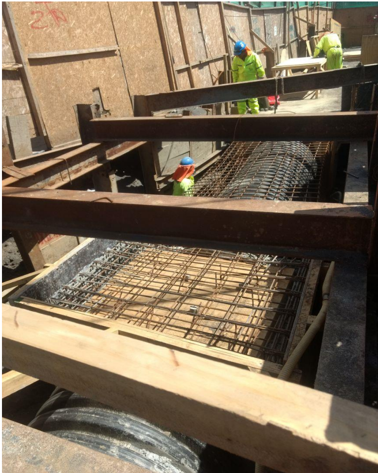
43 FIGURA 4-23 INSTALACION TUBO CORRUGADO (CALLE CAUPOLICAN)
