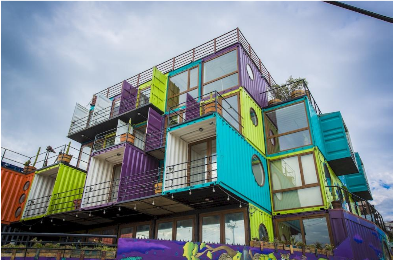
Figura 1-14. WineBox, Apart Hotel Valparaíso
