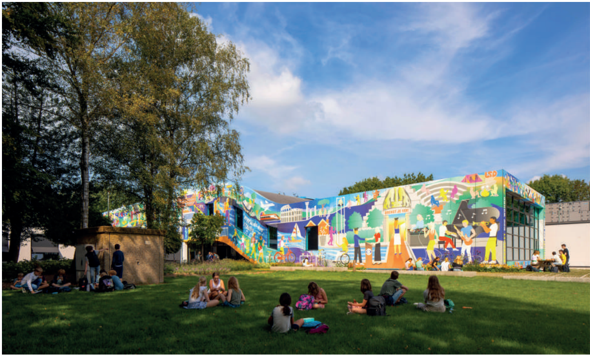
Fig59. "Gymnasium Beekvliet / MVRDV" https://www.archdaily.com/1007678/gymnasium-beekvliet-mvrdiv
