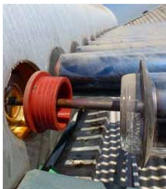
Figura 1-3 Tubos Heat pipe
