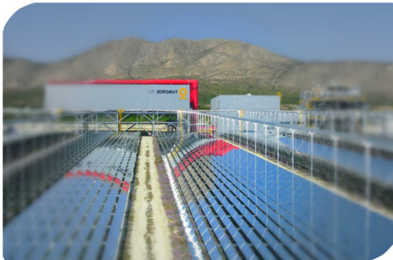
Figura 1.8: Colectores lineales Fresnel
