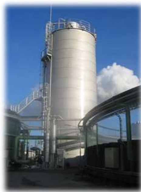
Figura 13 Reactor Upflow blanket (UASB) (C
