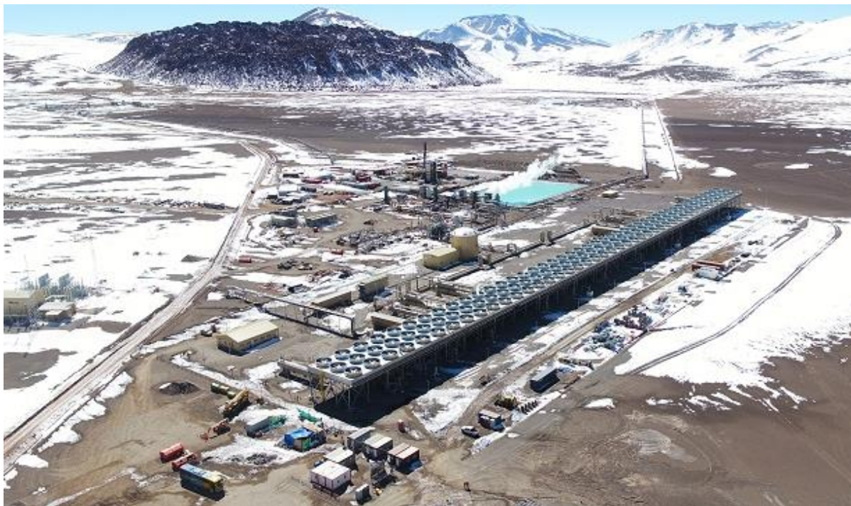
Figure 26: “Cerro Pabellón”, geothermal power plant in Ollague, Chile.
