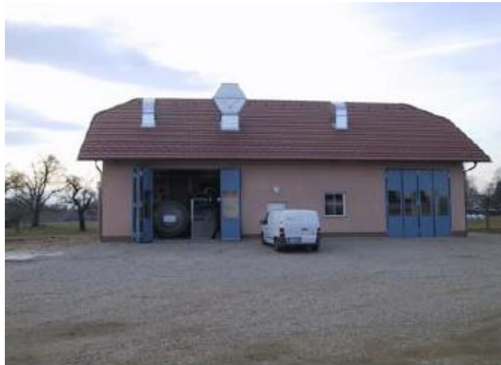
Figure 36: Power house of the ORC plant of the Altheim geothermal project [56]
