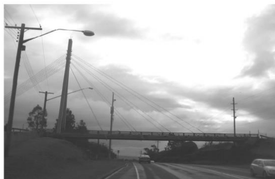
(b) UWS cable stayed bridge
