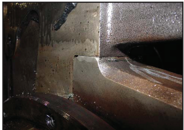
Figure 10 Add Charge Welded main caps
