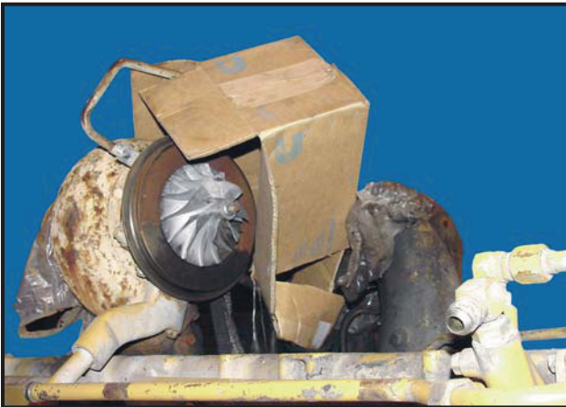
Figure 7 Add Charge Missing part – turbocharger compressor housing missing and improper protection from weather
