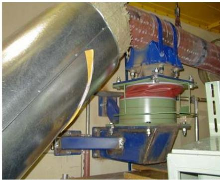
Fig. 8 VES damper at the RL76 in RB LO2 (damper's piston at the piping, housing at the RB wall)
