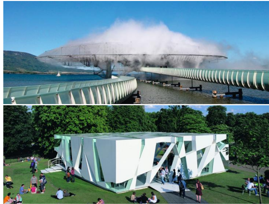
Fig. 13 "Blur Building" desde el exterior, Fuente: (Photography by Beat Widmer, Blur Building, s. f.)
