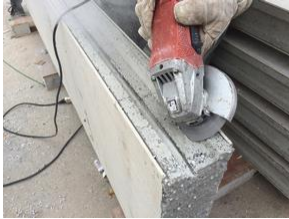
Figura 2-28 Corte de Panel Fast-Work
