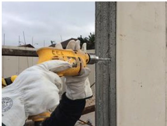
Figura 2-31 Perforaciones a Panel Fast-Work
