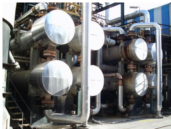
Figura IV.11: Vista angular C-1201
