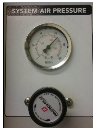
Figura 3-6: System Air Pressure.
