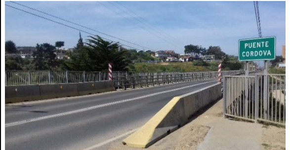
Figura 8-35 Vista general puente Córdoba
