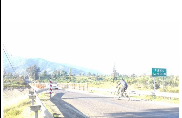
Figura 8-96 Vista general puente Illalolen
