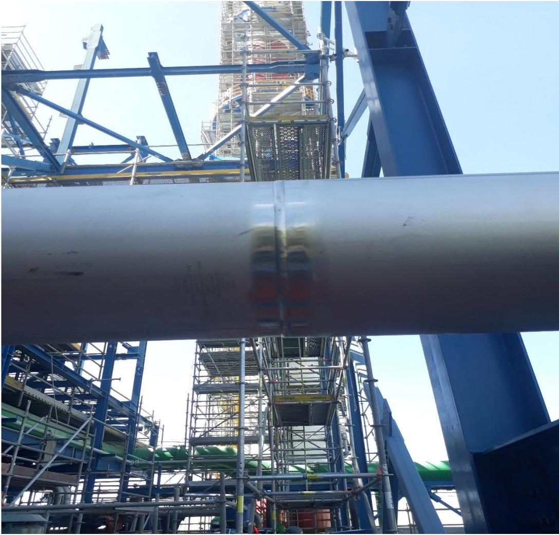
Figura 2-35 Unión BUTTWELD
